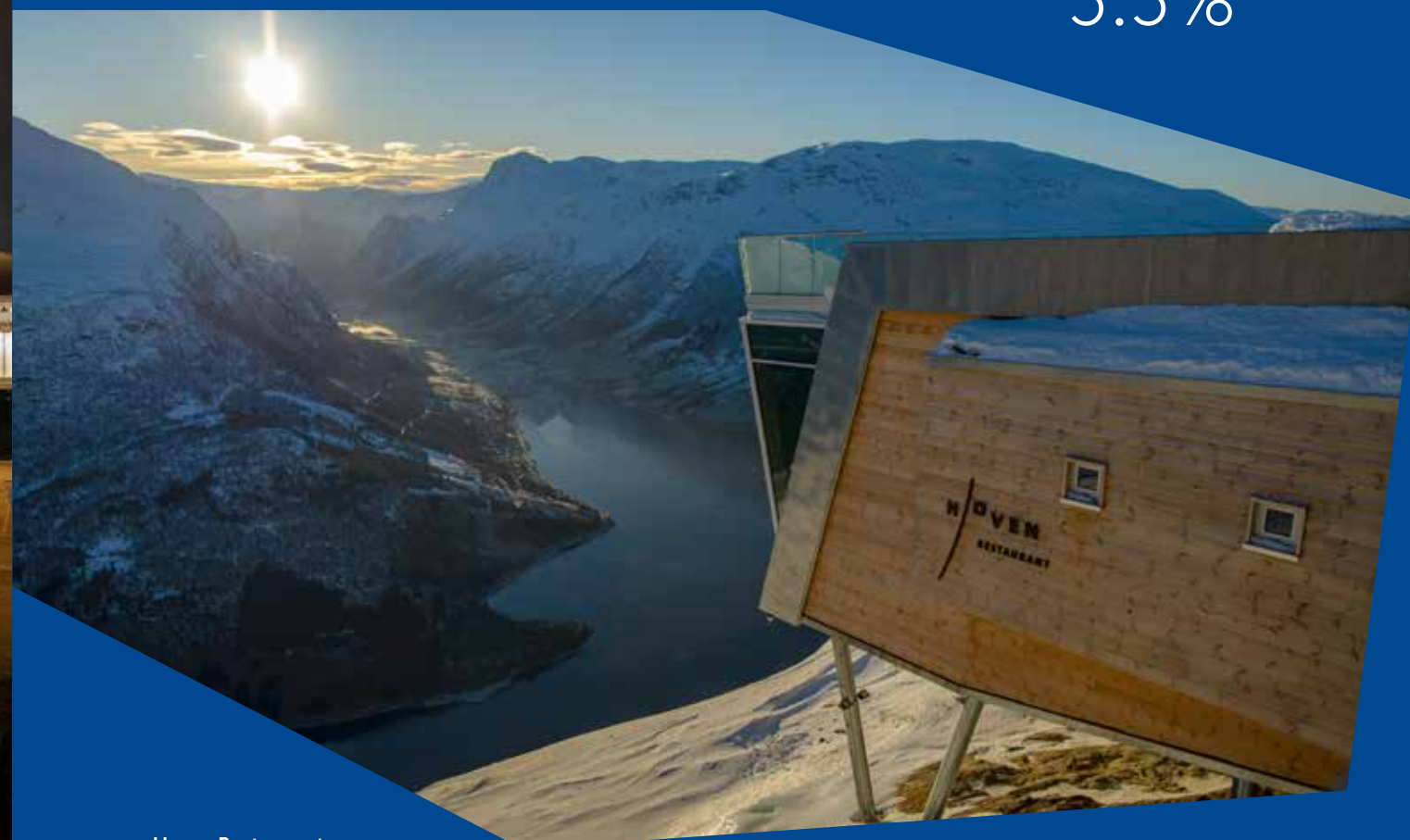
Hoven Restaurant Loen, Norway Roofing + Waterproofing Derbigum® SP4 FR; Derbigum® GC
